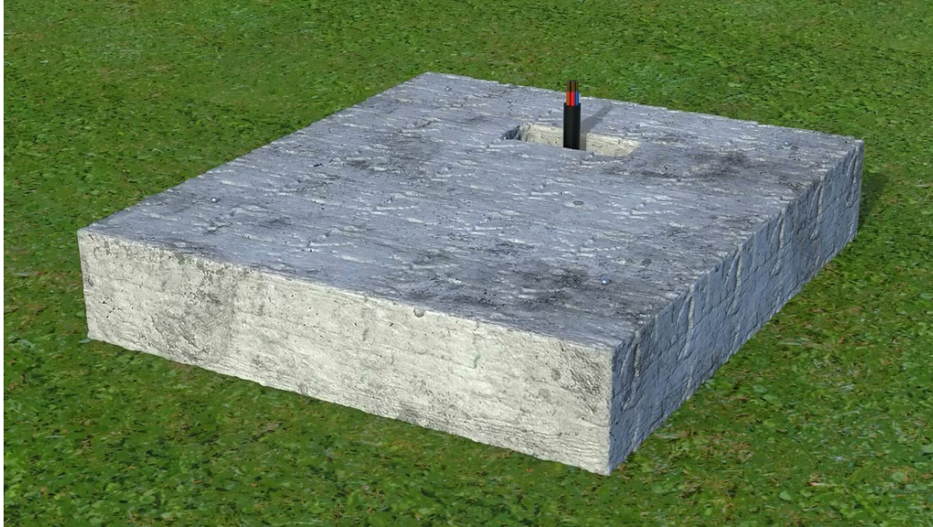
Fig. 3-1 Cabinet equipment cement foundation form
